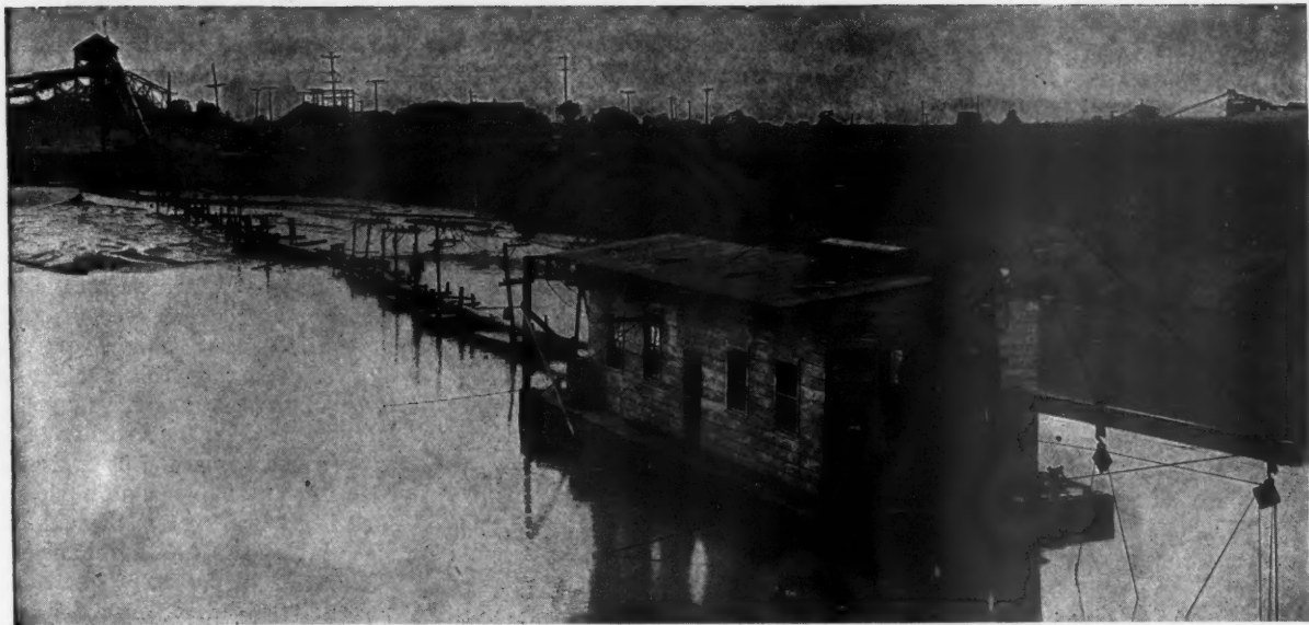
15-In Morris Dredge and Booster Pump delivering sand and gravel direct to screens. The booster pump is located in the first building on the bank
